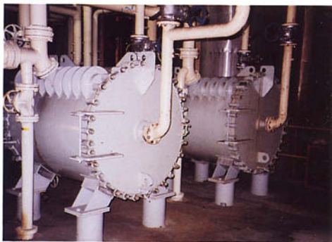
The three stage spiral heat exchanger at Lever Brothers Company, Hammond, Indiana, will perform as an upflow condenser with the condensate being removed between each stage.
