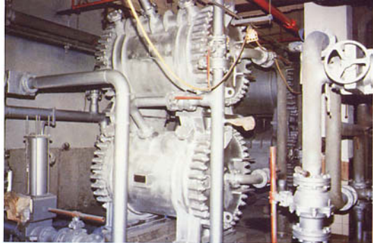
Four spiral heat exchangers at the Carver-Groenfield sludge dehydration plant at Los Angeles, California, recover heat in an oil slurry interchange between evaporative stages.
